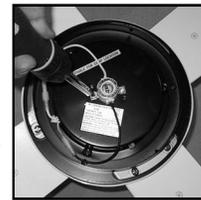
**(c)** Screw in lamp. Touch ceramic portion of lamp only, not glass.
