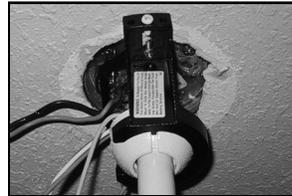
**(9)** Loosen set screws on the sides of the hanging bracket. Lift canopy to ceiling. With slots on side of canopy aligned with set screws on hanging bracket, tighten set screws to hold canopy in place.
