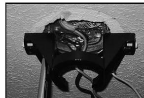
(3) Remove the stopper screw and loosen the set screw on the fan collar. Set the stopper screw aside for step (5).
