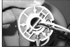
**(8)** Lift fan to ceiling and set half ball in the hanging bracket so that the ridge on the edge of the hanging bracket is seated in the slotted channel in the half ball.
